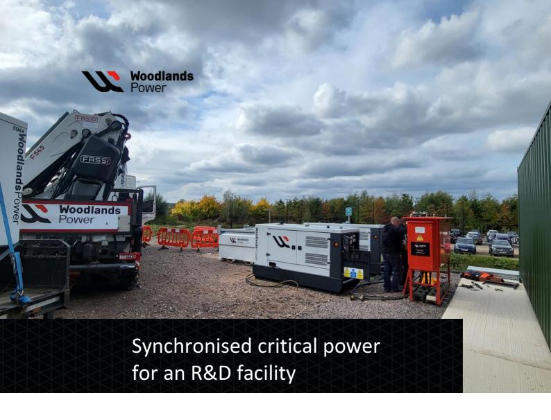
Our client required generators to support a critical load at an R&D facility while the mains supply was due for an upgrade.
